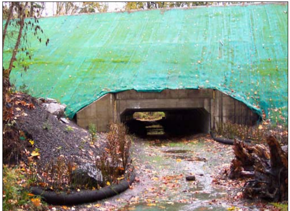
Water starts flowing through the new culvert.
