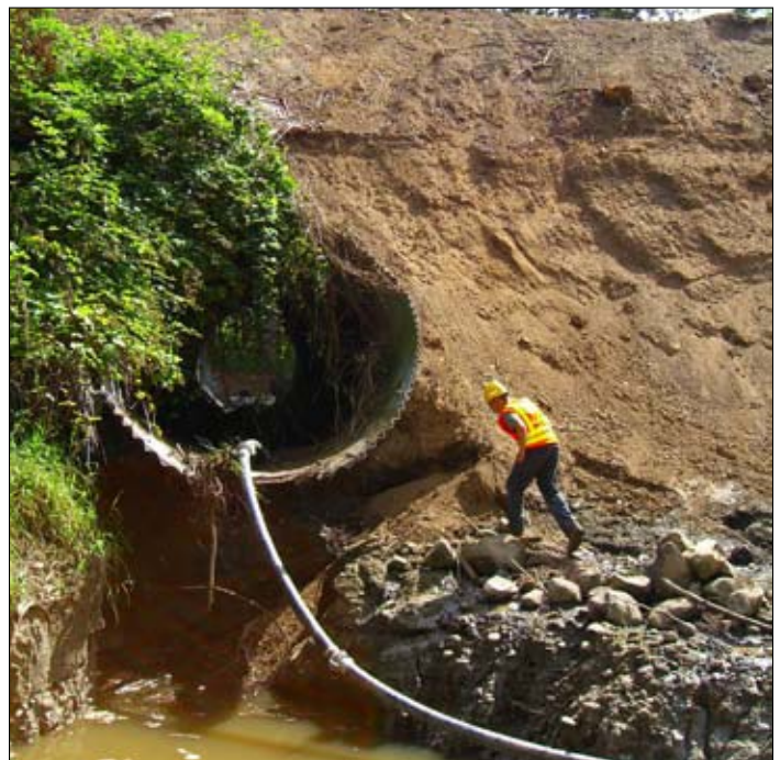
The old culvert sat high above the stream bed.
