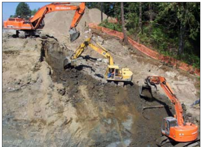
King sized bucket brigade: Crews worked in tight spaces and on steep slopes to conserve space and limit adverse effects to the surrounding area.
